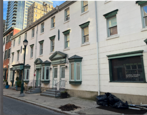
VIEW FROM SANSOM STREET
